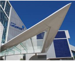
After the renovation of the city hall in Lelystad, the main entrance is marked by an inviting canopy with a fully glass roof. The canopy follows the contours of the building and seems to float above the building entrance. Ector Hoogstad Architecten, also responsible for the design of the original city hall in 1983, has challenged Octatube to realize an all glass roof.
