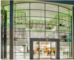
ABN Amro's new regional head office is featured by a fully glazed and bent entrance façade. The entrance is situated at the Koningskade, directly visible for everybody entering the city of The Hague by car. They notice the façade has a green hue, which has been processed in the glass upon special request from the client.
